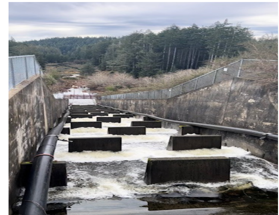
Spillway at Upper Pony Creek
