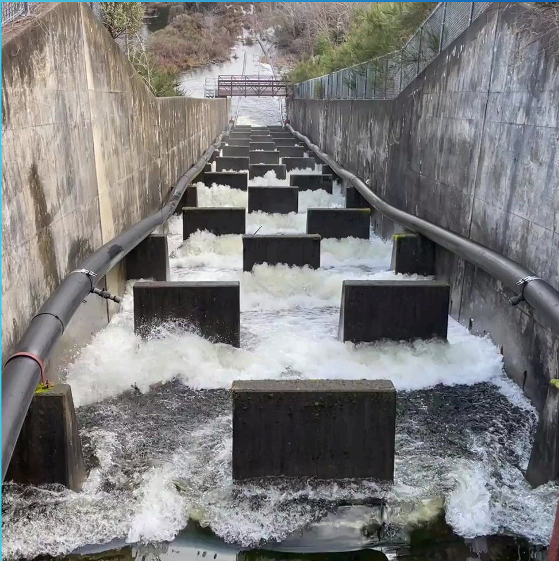
Spillway at Upper Pony Creek Reservoir
