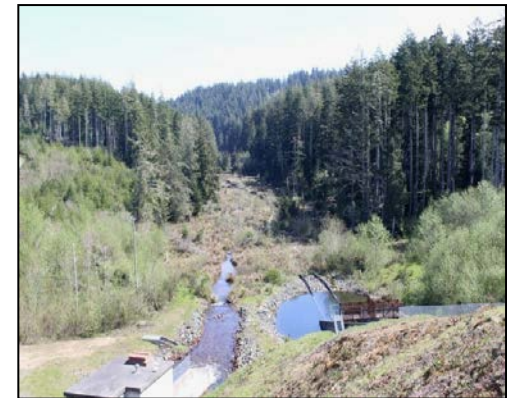
Spillway at Upper Pony Creek
