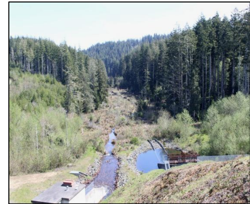
Spillway at Upper Pony Creek
