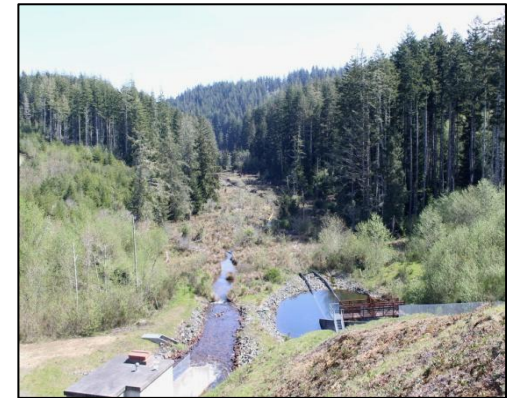
Spillway at Upper Pony Creek
