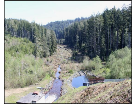
Spillway at Upper Pony Creek
