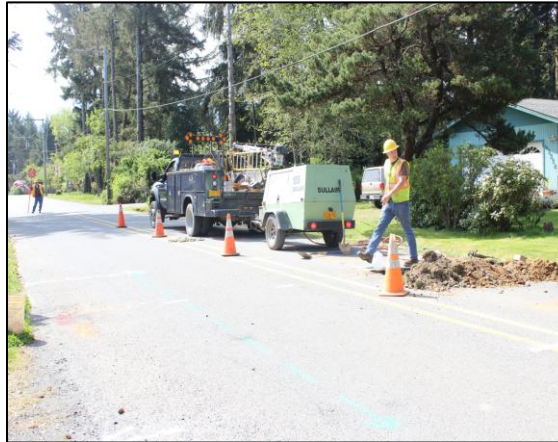
Crew members installing a new service
