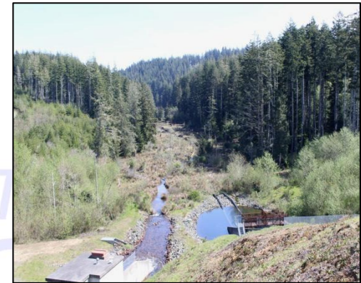
Spillway at Upper Pony Creek
