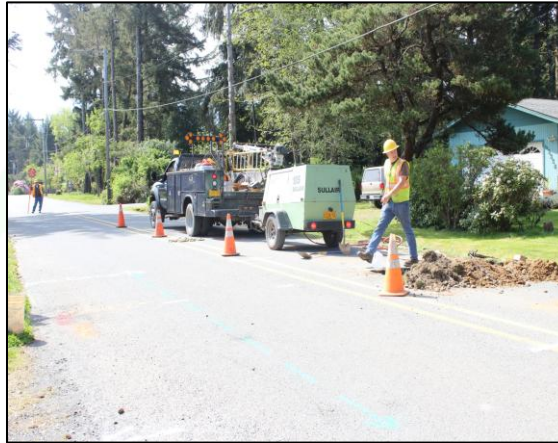
Crew members installing a new service
